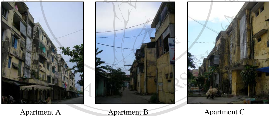
Figure 1-4: Three Buildings of Dong Da apartment Complex in Hue, Vietnam (2007)
